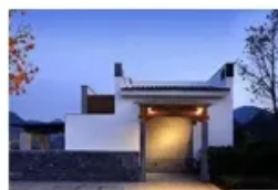
Household Energy Storage
