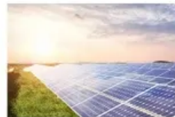
Energy Storage System
