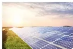
Energy Storage System
